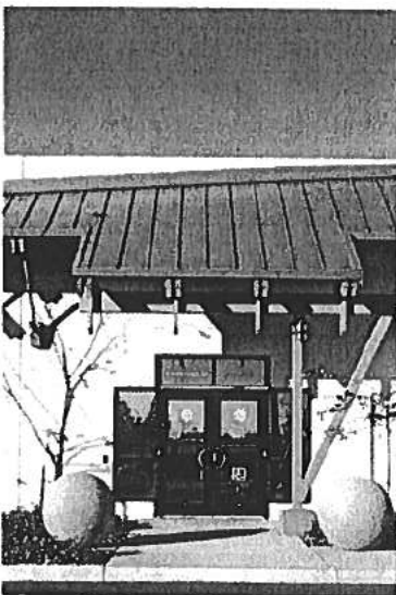
view at building entry
